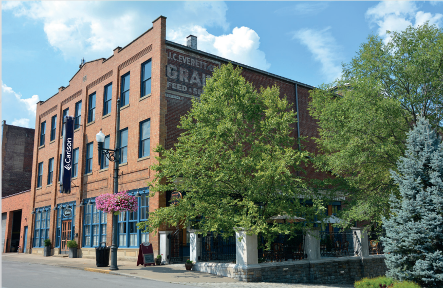
Carlson Headquarters, Maysville, Kentucky USA
