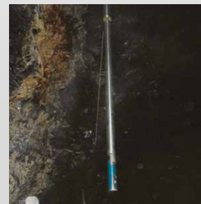
The C-ALS system deployed downhole to survey an inaccessible underground void.
